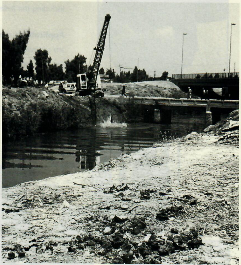
December 1995: UNSCOM directs the dredging of the Tigris River.
